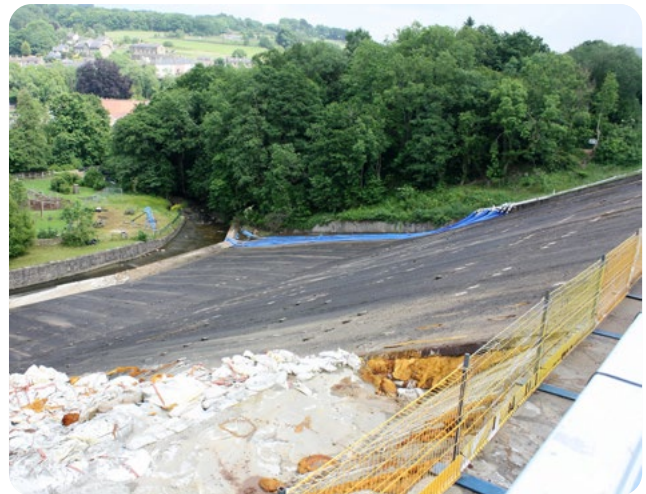
The current auxiliary spillway, which will be de-commissioned and grassed over.
