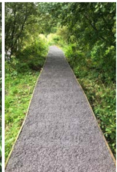
After: Improved footpath
