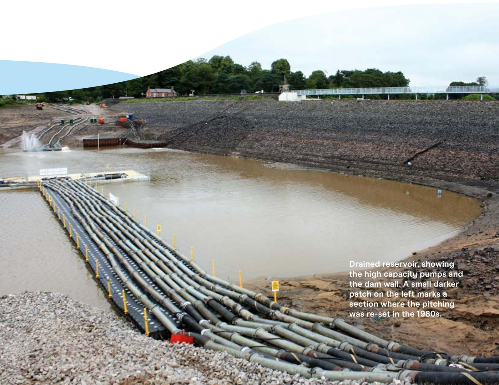
Drained reservoir, showing the high capacity pumps and the dam wall. A small darker patch on the left marks a section where the pitching was re-set in the 1980s.
