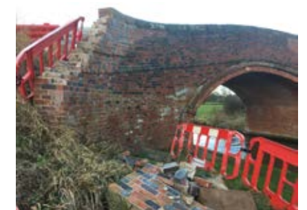
Above: Golden Nook Bridge vehicle damage
