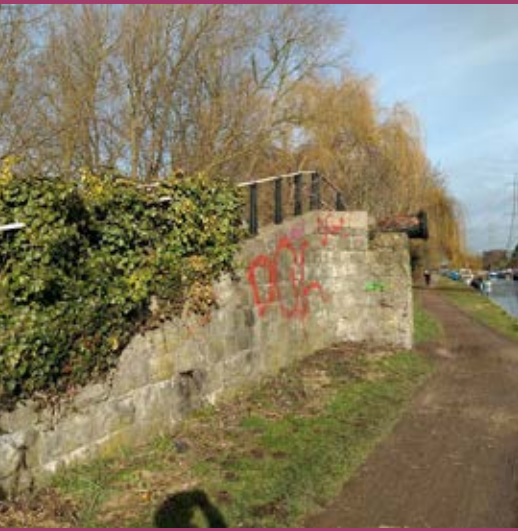
Stone bridge and towpath, Enfield Lock Image: Clare Moloney
