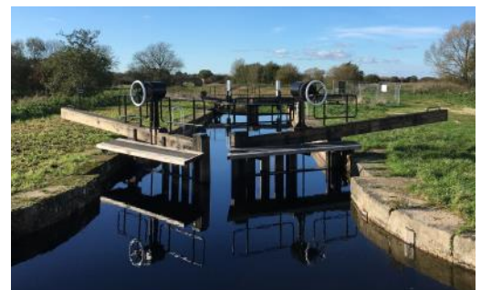
Top to bottom: Dredging (credit Malcolm Slater), Tree works underway, newly restored Thornton Lock.
