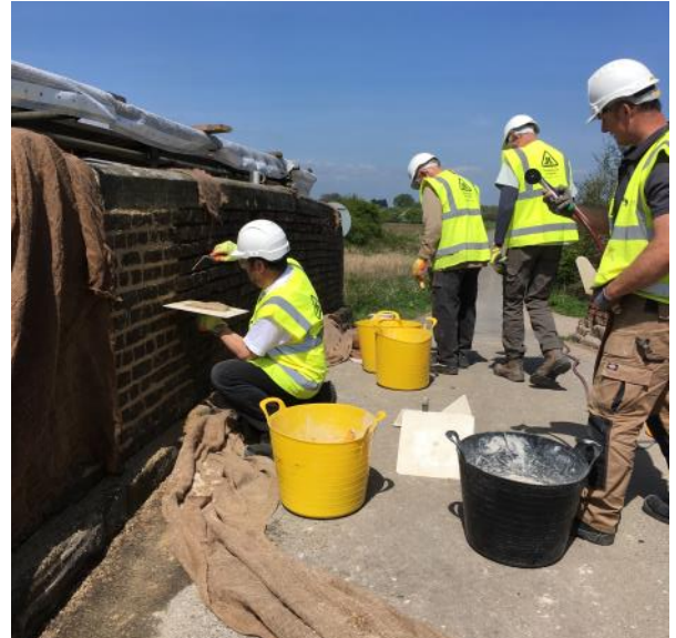
Above: volunteers working during the road closure; Below (L to R): Brickwork before work started; A section of damaged brickwork removed; the newly repointed inner parapet wall.
