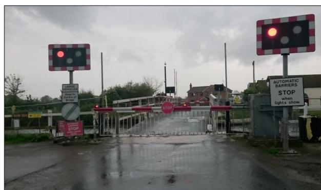
*Sandfield Bridge showing poor sight of oncoming vehicles over the bridge, no hatching and adjoining track junction on left*
