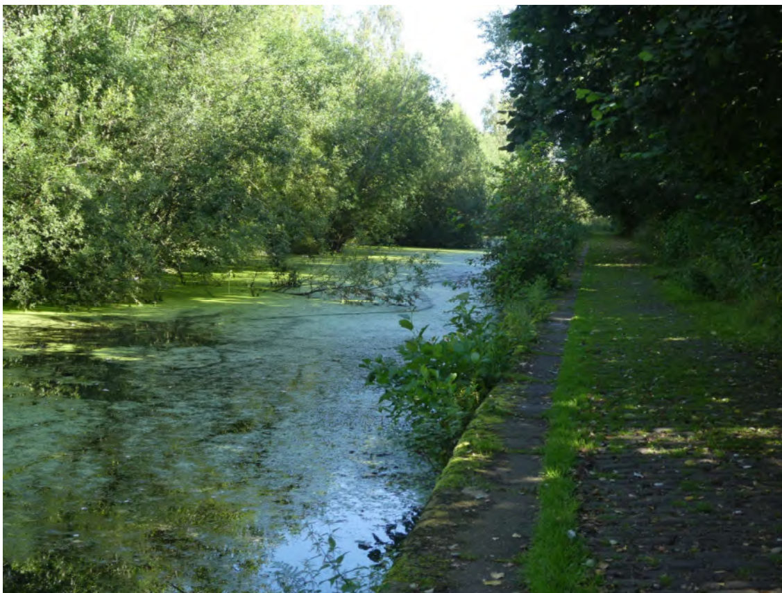
Photograph 1 - Trees encroaching across canal at Radcliffe
