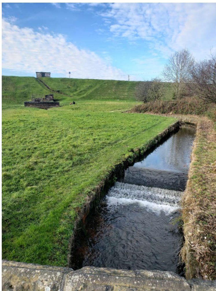
Photograph 2 – Canal Feeder looking toward Elton Reservoir
