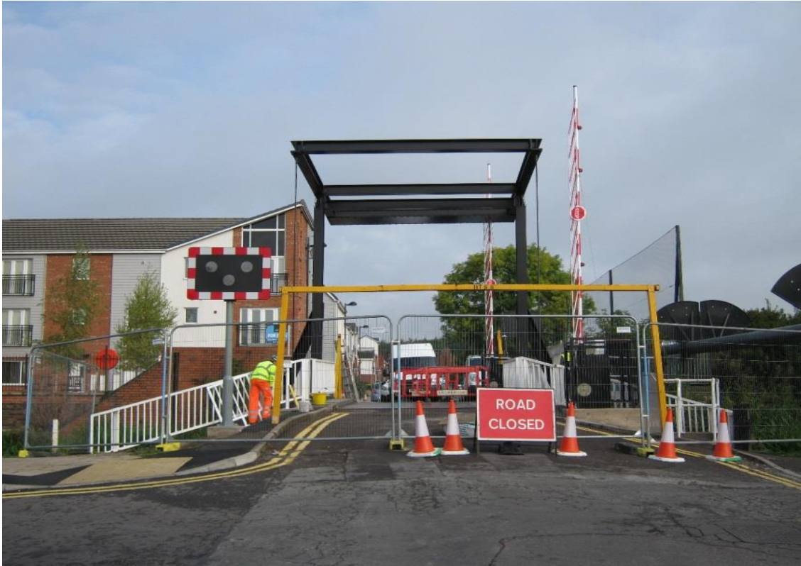
Ivy House Lift Bridge, Caldon Canal undergoing safety improvement works
