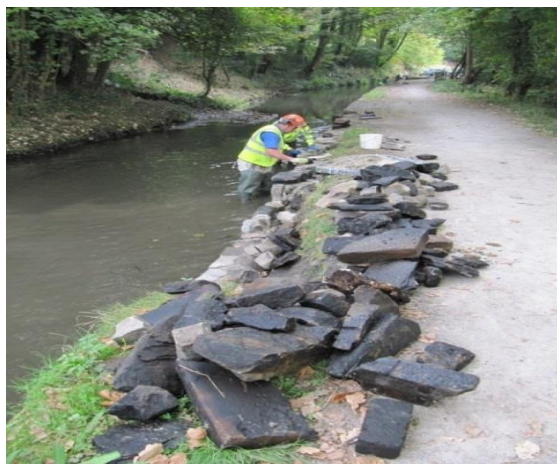
Swansea canal – Waterway wall repairs
