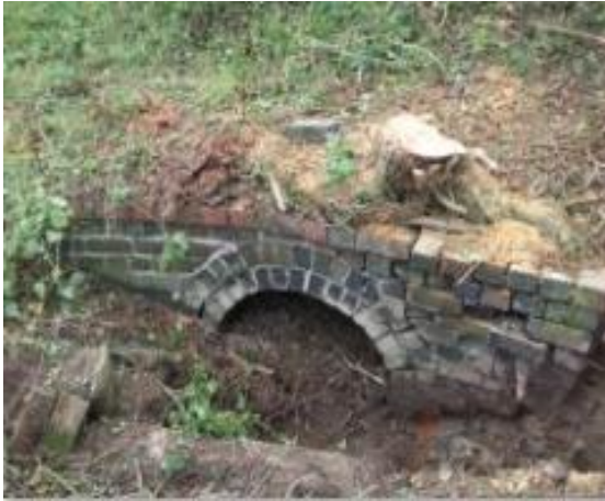
Culvert repair Montgomery Canal – before/after
