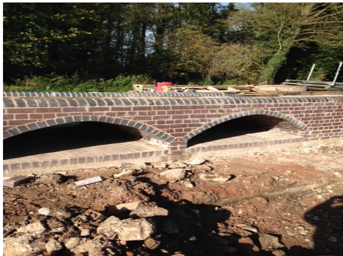
South Stratford Canal - Weir rebuild
