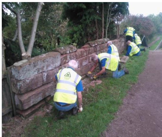
Worcester area parapet wall repairs
