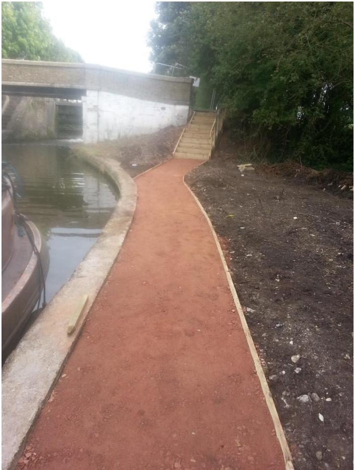
Mooring improvements Grand Union Canal, Rickmansworth
