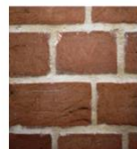
High quality, flush jointed repointing
