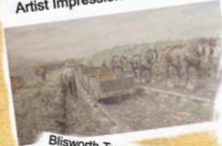
Blisworth Tunnel showing the Horse Boat Road and Tramway
