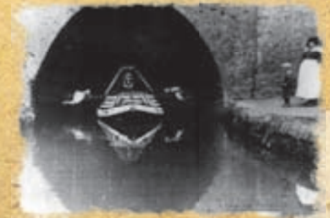
Men legging through the South Portal of Blisworth Tunnel
