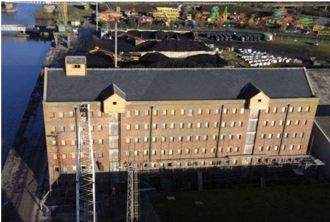
Figure 3. North Warehouse, Sharpness was repaired in 2012/13 and is no longer a Building at Risk.
