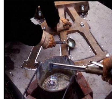
Traditional lead pouring on lock gate anchor frame
