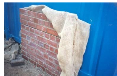
A sample panel for lime mortar in brick repairs
