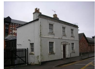
Lime rendered bridgekeepers cottage before repainting
