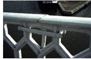
An early strap repair to a cracked cast iron handrail
