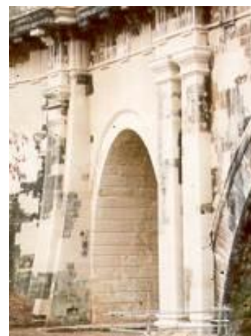
Lime washed flood arch of restored aqueduct
