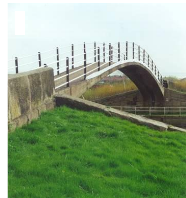
Reinforced concrete footbridge, River Trent, 1915. Listed grade II*
