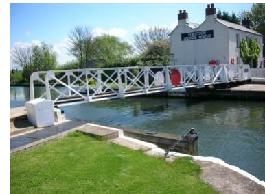
Steel swing bridge
