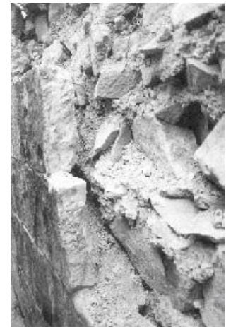
Disintegrating core work
