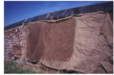
Protecting with wet hessian
