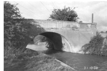
A cement rendered bridge
