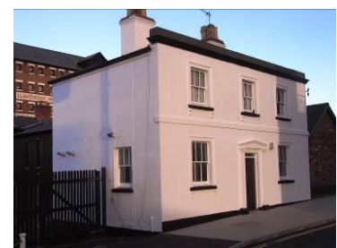
Cottage after repainting with a mineral paint
