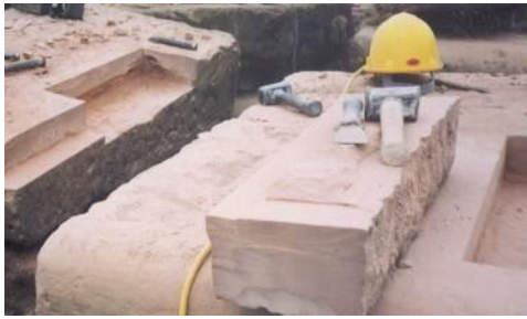
Preparation for piecing-in
