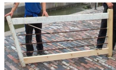
Repaired towpath 'clapper' gate before repainting
