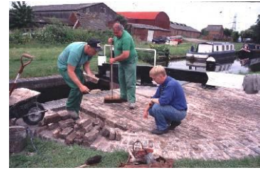
Replacing brickwork on a historic heel grip platform.
