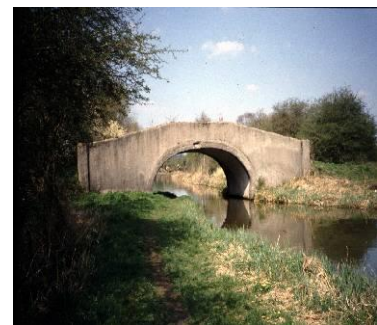
A 'gunited' bridge. Such drastic action has little to do with conservation
