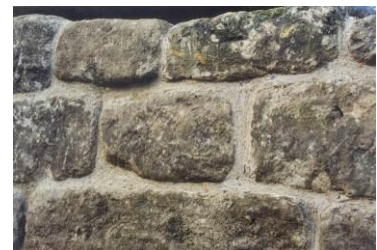
Good pointing employing a lime mortar
