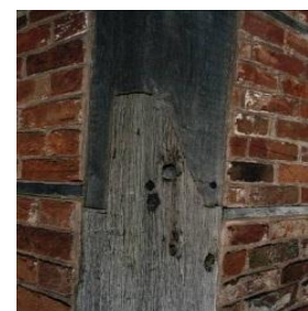
A traditional scarf joint repair to a corner post
