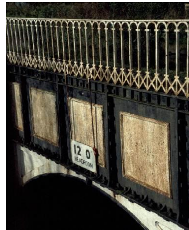
Old paint systems must be removed with care
