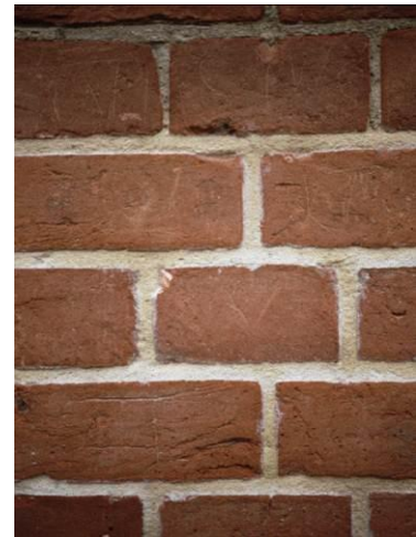
Good quality traditional brickwork
