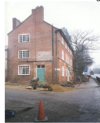
After cleaning with a mildly abrasive system
