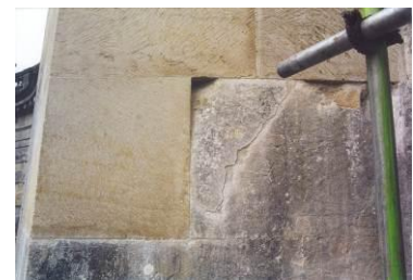
The strength of new stones must match that of old ones
