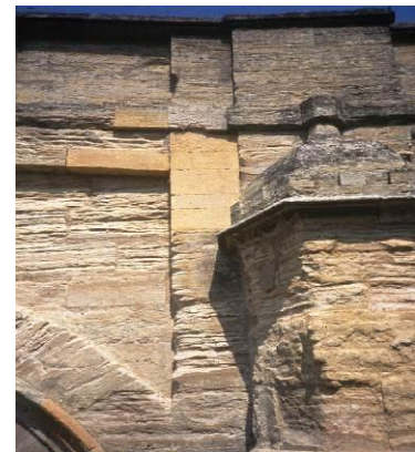
Replacement with new stone
