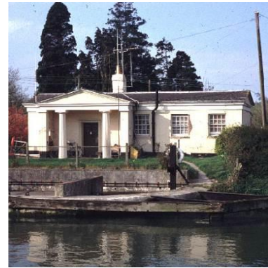
Paint is traditional for some waterway buildings
