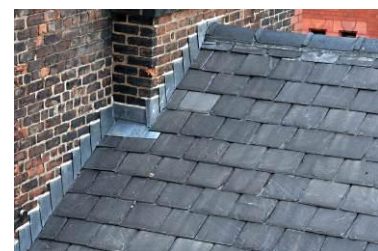
Lead flashings on a roof
