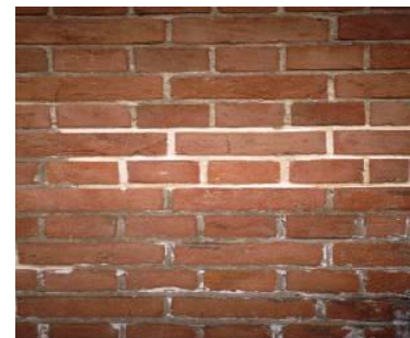
Lime based mortar (white) and cement based mortar (grey) in the same wall
