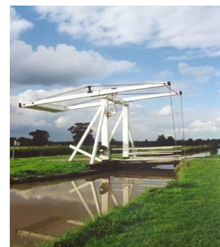
Traditional carpentry is still found in operational structures.
