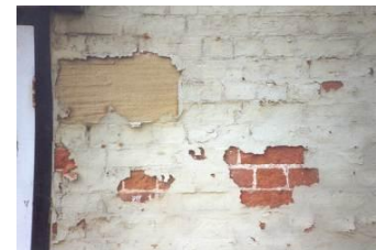
Results of applying plastic-based paint to historic brickwork
