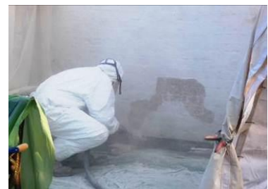
Removing masonry paint by sympathetic blast cleaning before repainting
