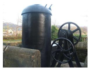
The bridge is made of iron girders with planking over the central section of the roadway. It is raised in the horizontal position via chain pulleys carried on an iron box-framed gantry, with the machinery contained in small compounds on the west bank. This consists of two large domed cylindrical counterweights each bearing the date 1865, the now redundant 19<sup>th</sup> century hand-crank and winch gear and 20<sup>th</sup> century metal boxes containing the electrical equipment.
