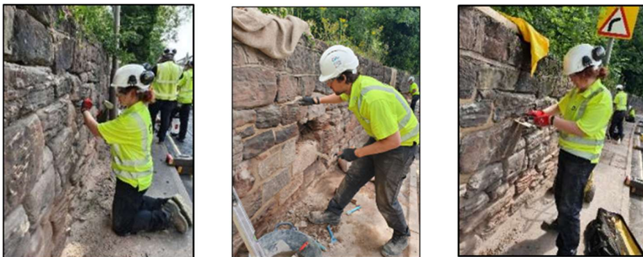
Apprentices undertaking boundary wall repairs
