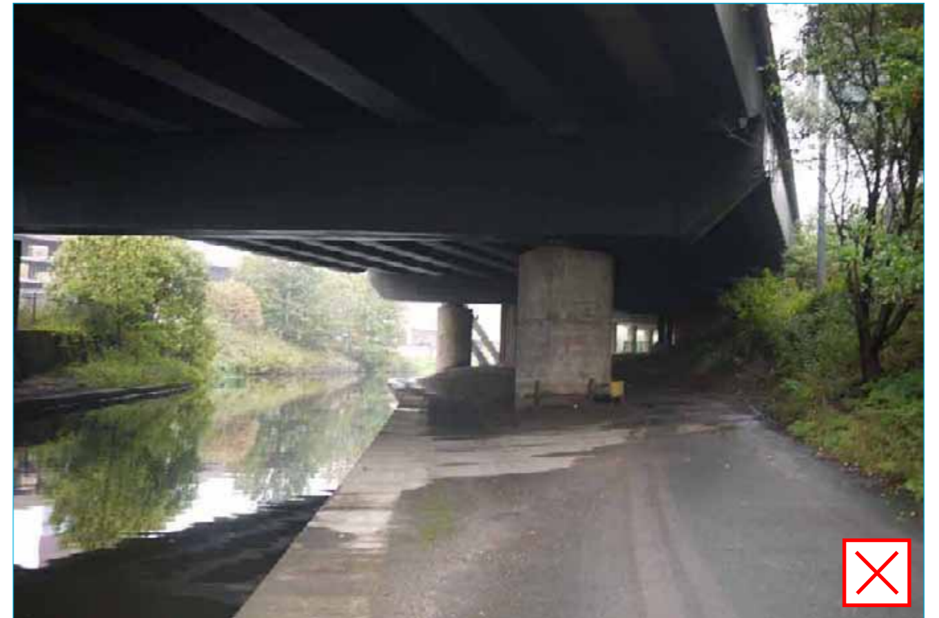
Fig.B2.1 - Bridge with a poor relationship with the canal below
