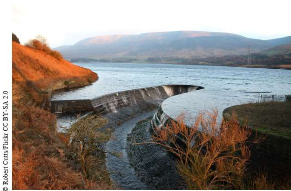
Figure 11: Example of bathtub spillway within reservoir
