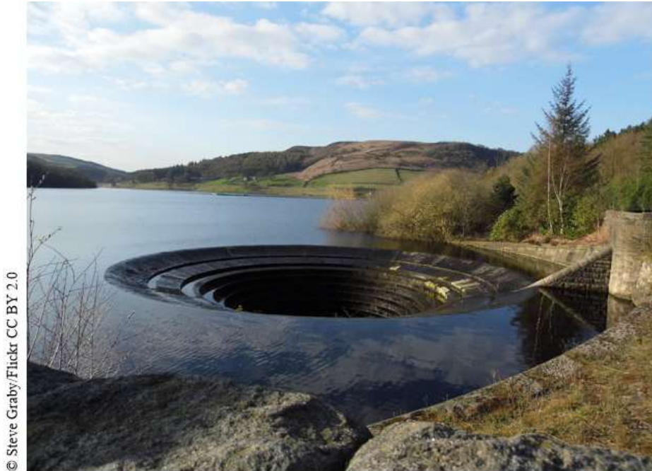
Figure 5: Example of Shaft Spillway Overflow within reservoir
