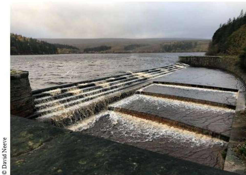
Figure 7: Example of a side channel spillway
