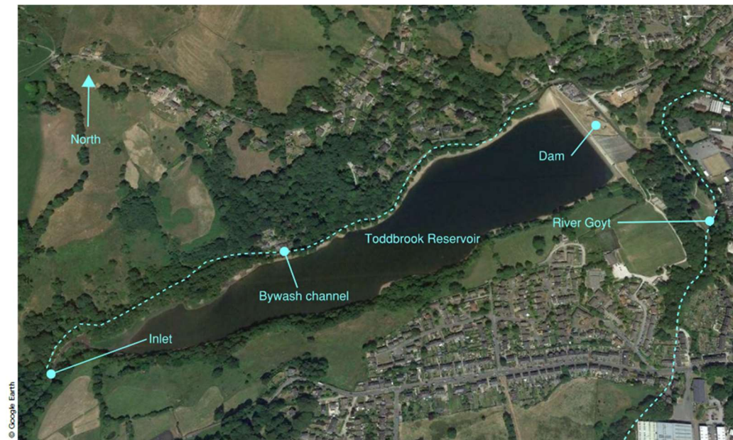
Figure 1. Toddbrook Reservoir key features
