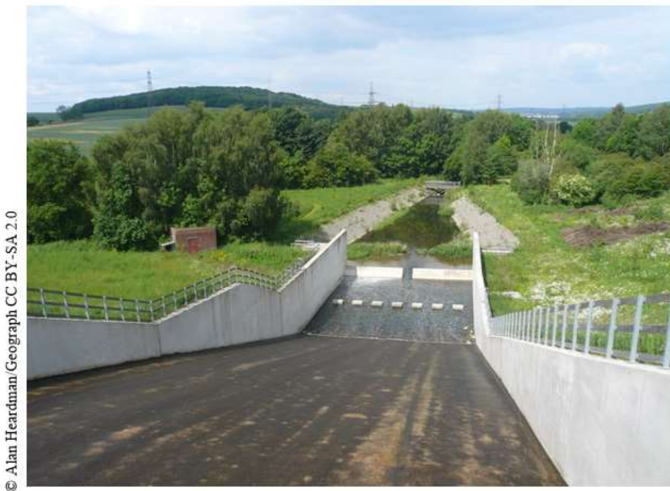
Figure 10: Example of a spillway located on a dam, with stilling basin at the downstream end
