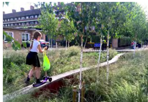
Joyce Square, Community Rainpark, Robert Bray Associates, 2017. Swales to convey and filter run-off, with secondary play paths
