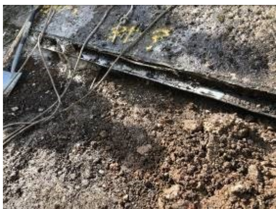
Water bar at joint
