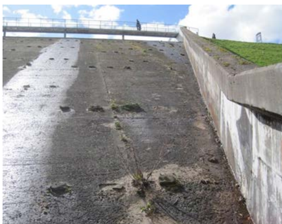
Flow from the top of the spillway
