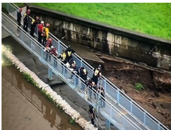
Damage at left hand end
