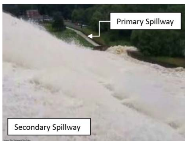
Flood event – 31 st July 2019
