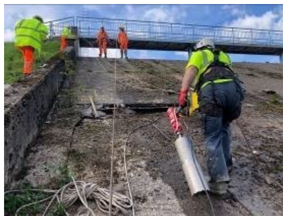
Excavation on the slope
