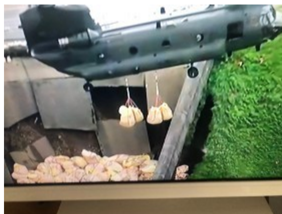
Emergency works (note the void outside the wall)
