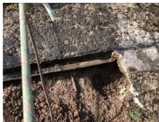
Excavation showing dowels and water bar
