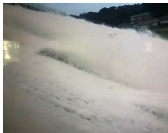
Flow on spillway channel
