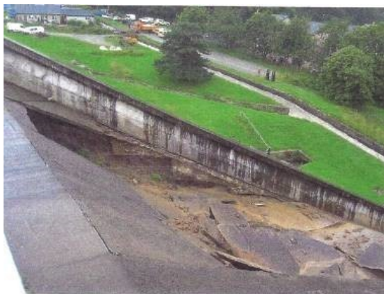
Shallow foundation to the left-hand wall
