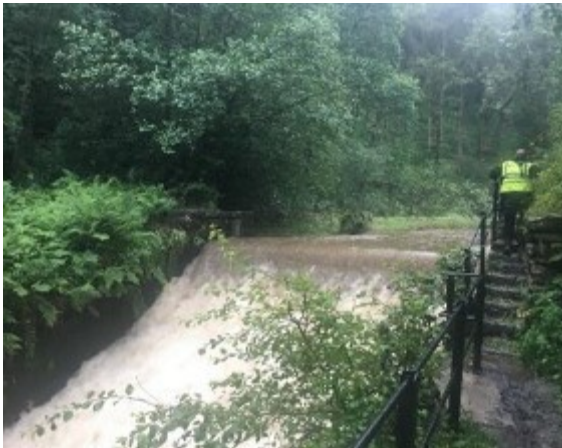
Inlet weir to bywash channel
