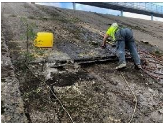
Excavation on the slope
