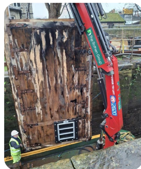
Above: Brighouse Lock, Calder & Hebble Navigation
