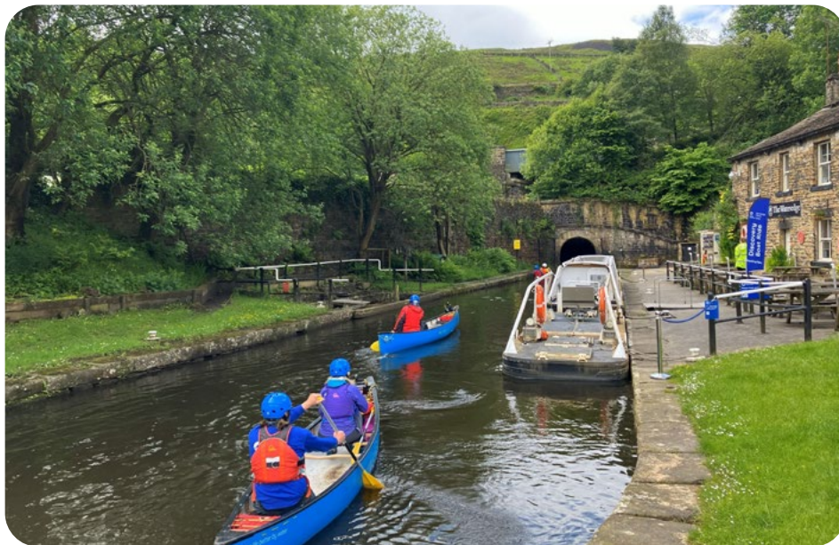
Left: Standedge Tunnel, Marsden, Huddersfield Narrow Canal
