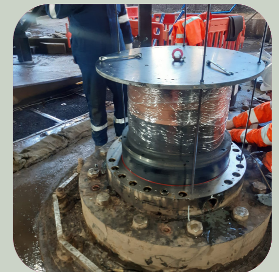
Changing the bearings and seals on one of the main cylinders
