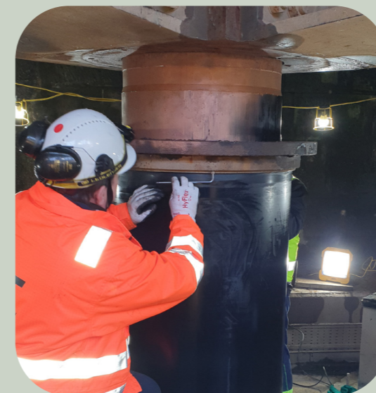
Removing main cylinder from bottom of caisson
