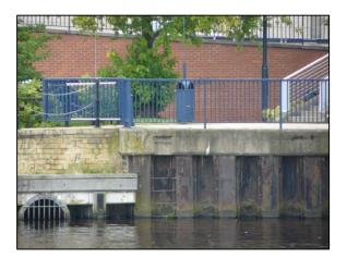
**Description** - Various types of wall construction with occasional fencing above. Ladders intended for emergency egress only access may be difficult, condition of ladders and fencing unknown.
