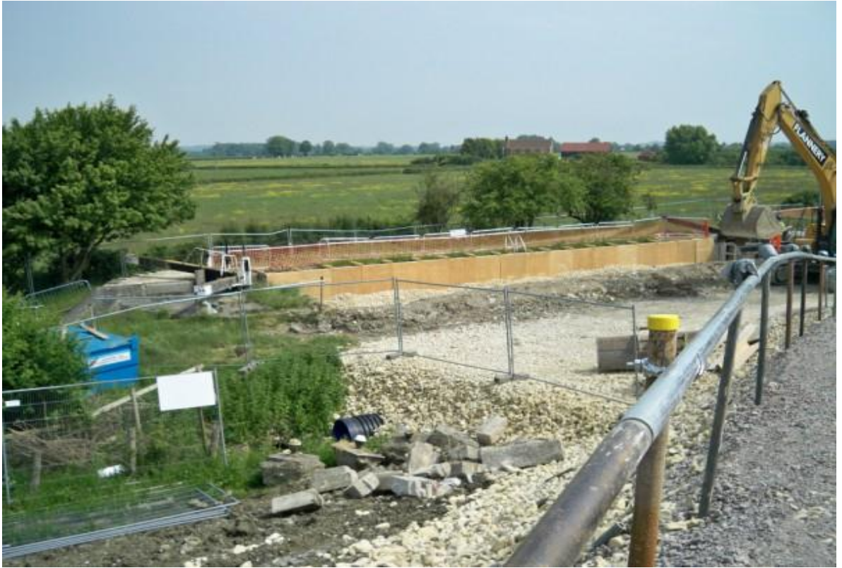
Lock 12 - Aylesbury Arm Emergency Repair Underway
