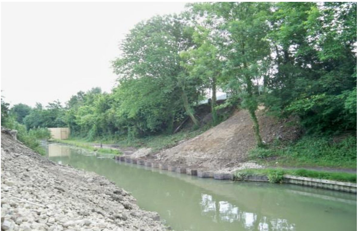
Reed Bridge, Slough Arm Emergency Project – Bridge Removed, Navigation Re-opened
