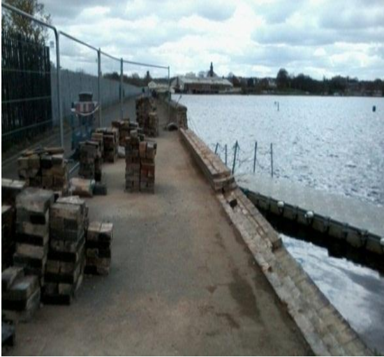
Photo showing the lowered dam wall
