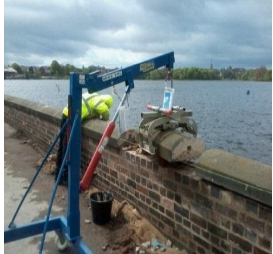
Lifting device placing the copings on wall
