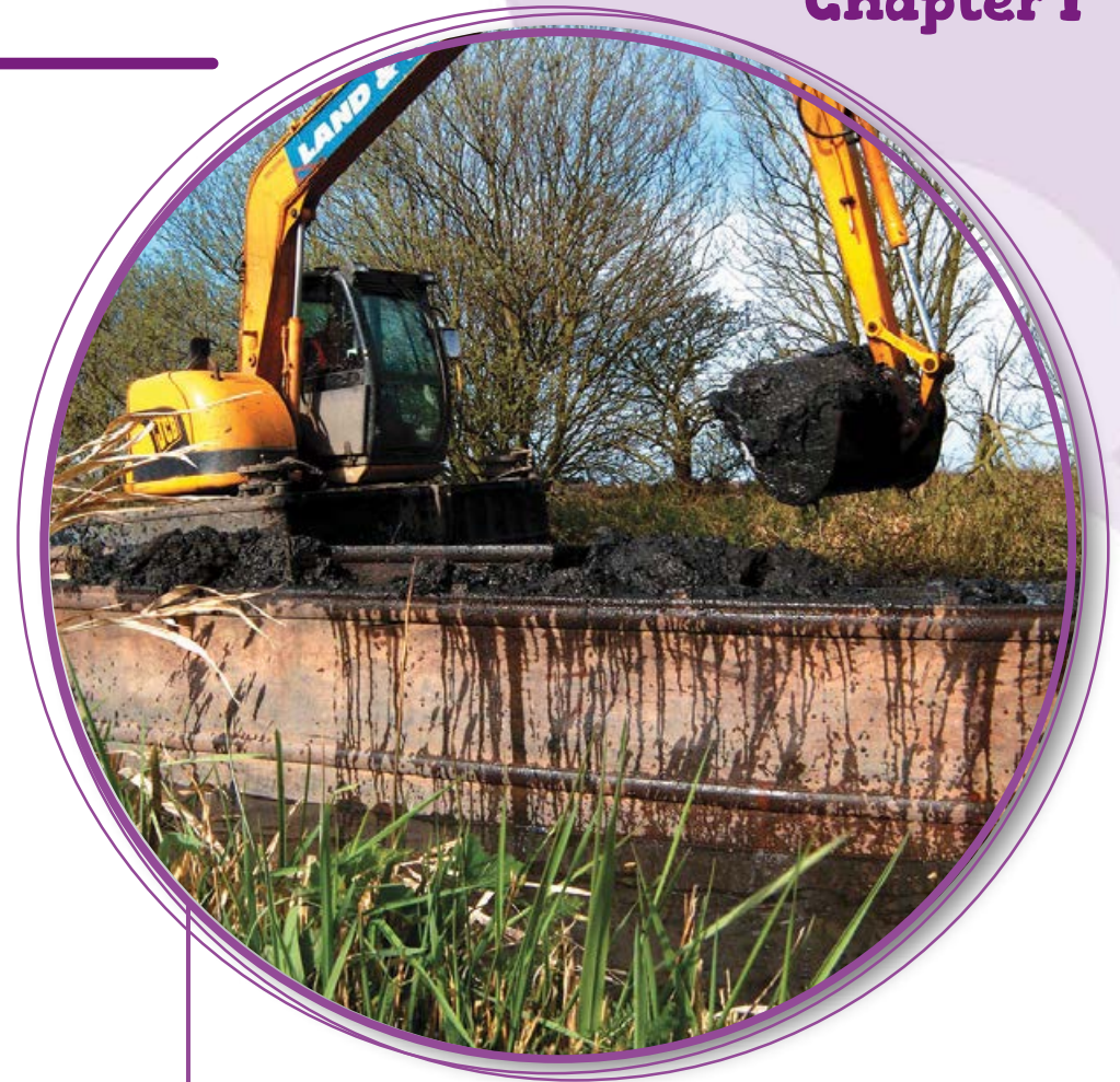
A dredger at work on the Birmingham & Fazeley Canal
