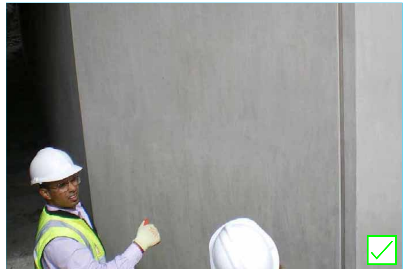
Fig.B15.2 - Well detailed, uniform concrete creates a high-quality environment
