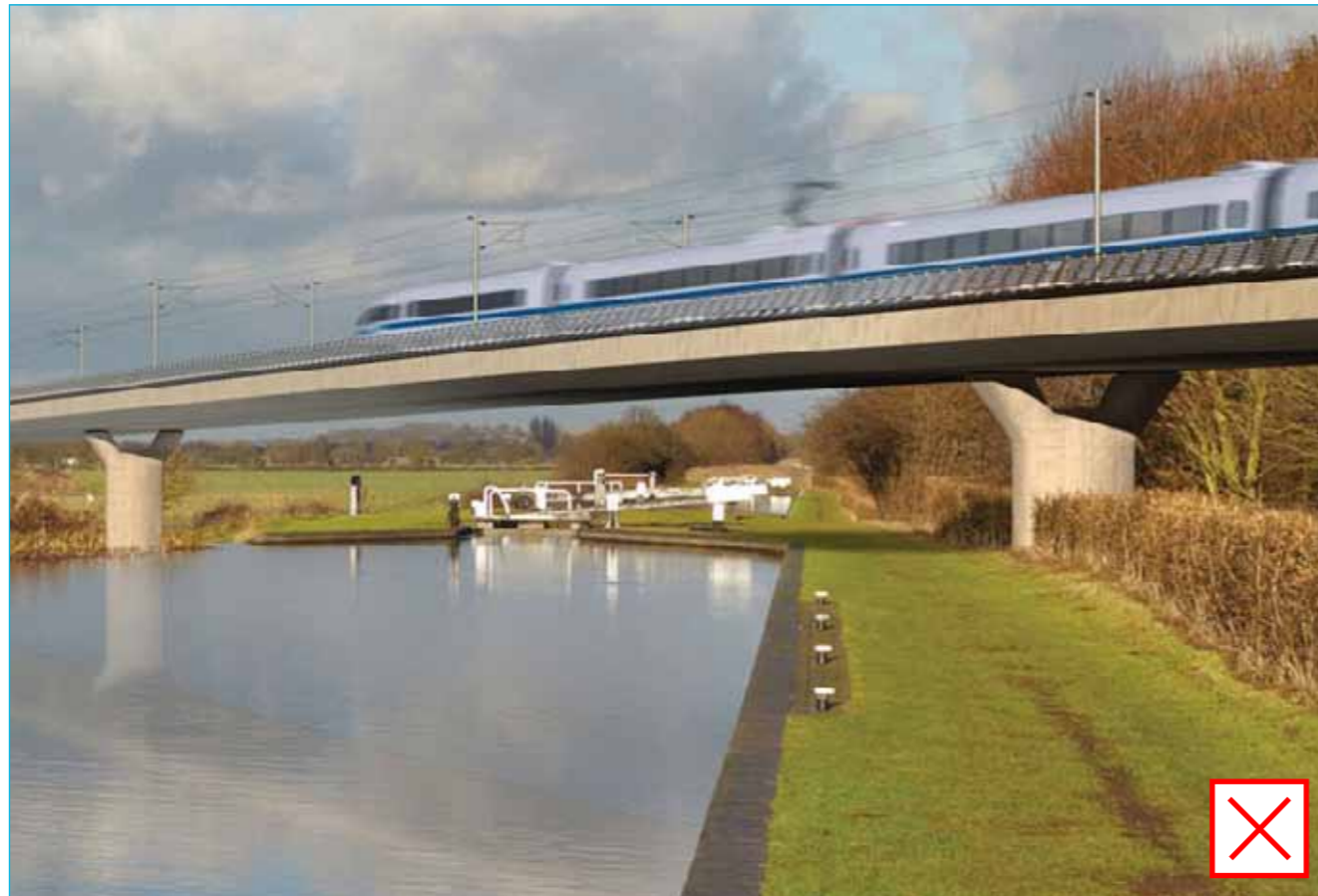
Fig.B7.3 - Piers aligned to the rail appear heavy and obtrusive from the towpath
