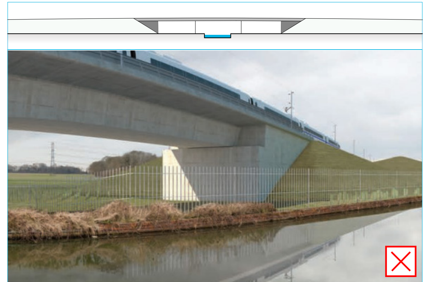
Fig.B5.9 - Vertical concrete abutment is an obvious intrusion into the landscape
