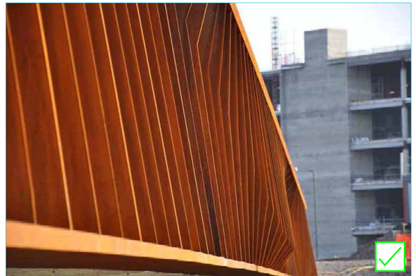
Fig.B15.4 - Weathering steel can form a positive element of a pedestrian environment
