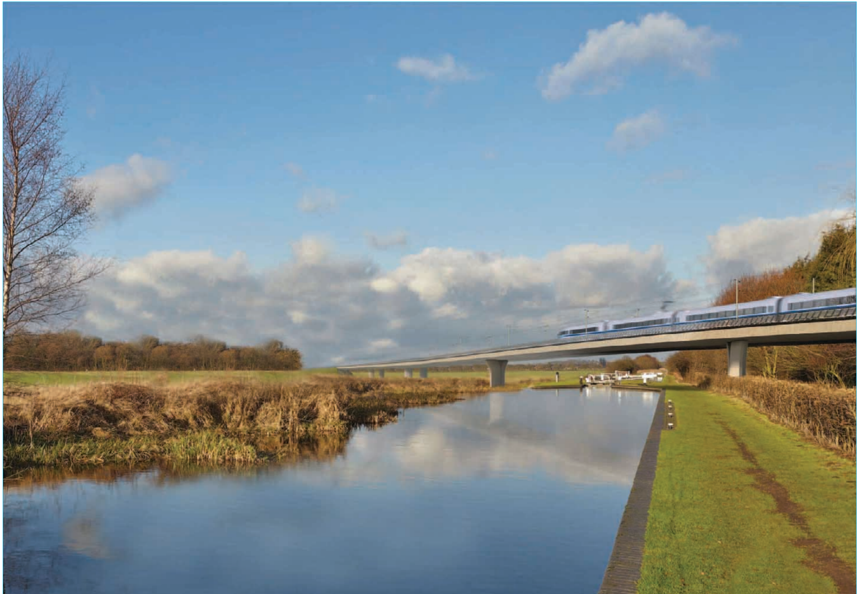
Fig.B5.11 - Sloped abutment face and multiple back-spans reduces negative visual impact and maintains open views
