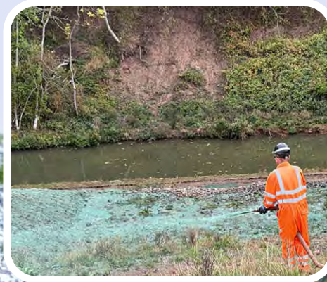
Inset: By spraying the slope with a 'soup of seeds' native plants will grow back and help bind the slope together
