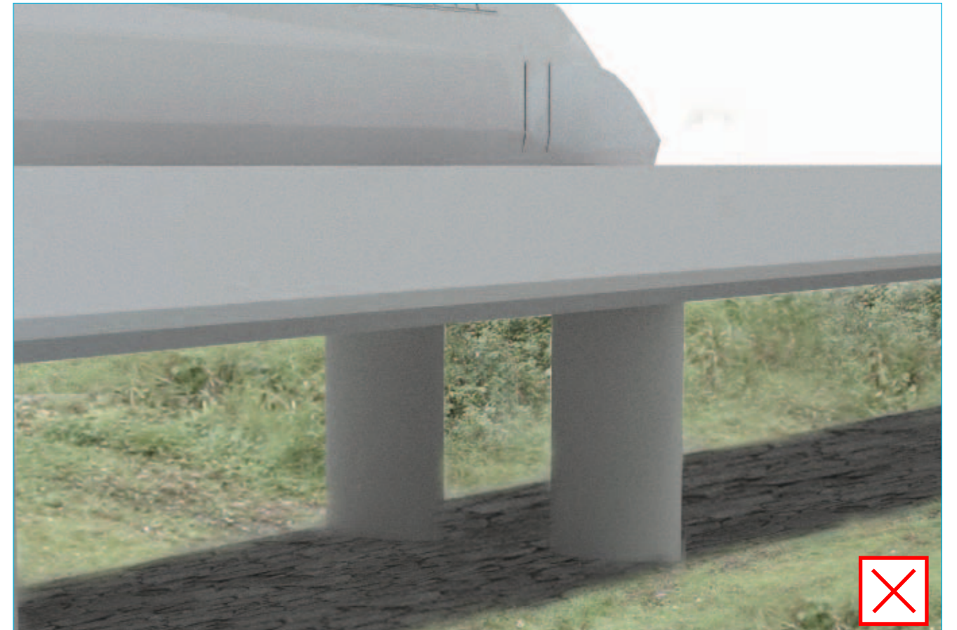
Fig.B13.3 - Large areas of abutment appear unsightly
