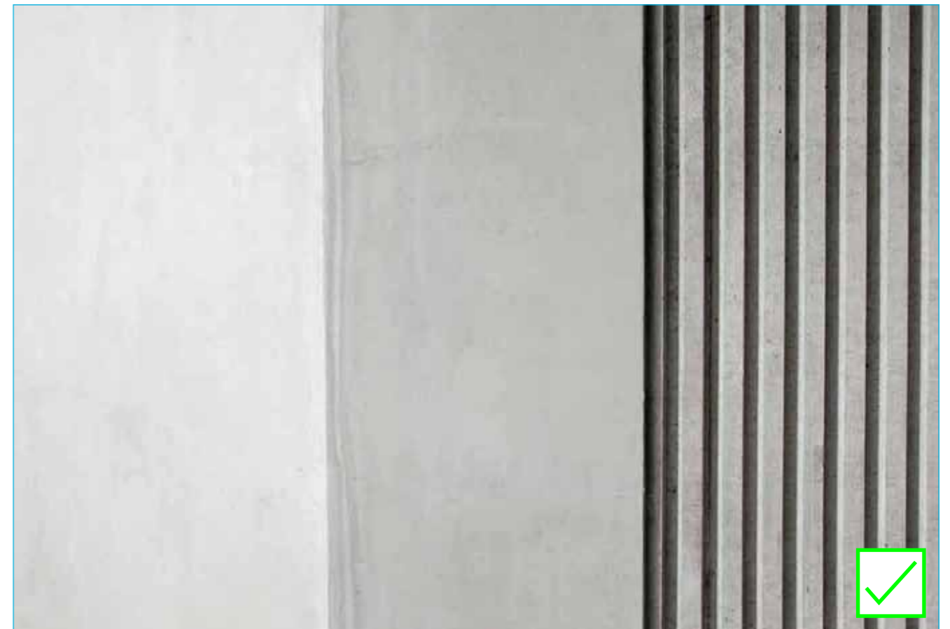
Fig.B15.3 - Textures and shadow gaps mask joints and reduce visual mass of concrete
