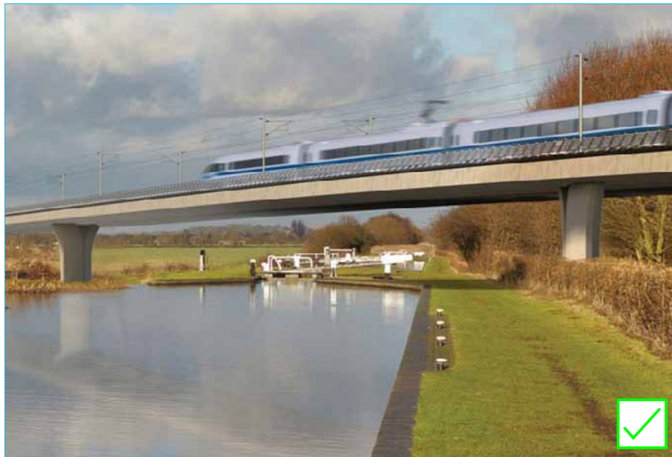
Fig.B7.4 - Piers aligned to the canal appear more slender from the towpath
