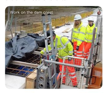
A protective, waterproof nib (short wall) has been added to the crest of the dam wall above the damaged spillway. This reaches down to create a seal with the dam's clay core and ensures no water from inside the reservoir can penetrate beneath the concrete slabs at the top of the spillway.
