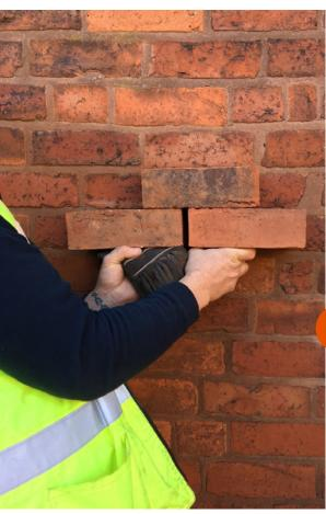
Many of the bricks at the Roundhouse were in poor condition and needed to be replaced. Because the Roundhouse is a Grade 2 listed building, we needed help from a special restoration team who were experienced in historic brickwork.
