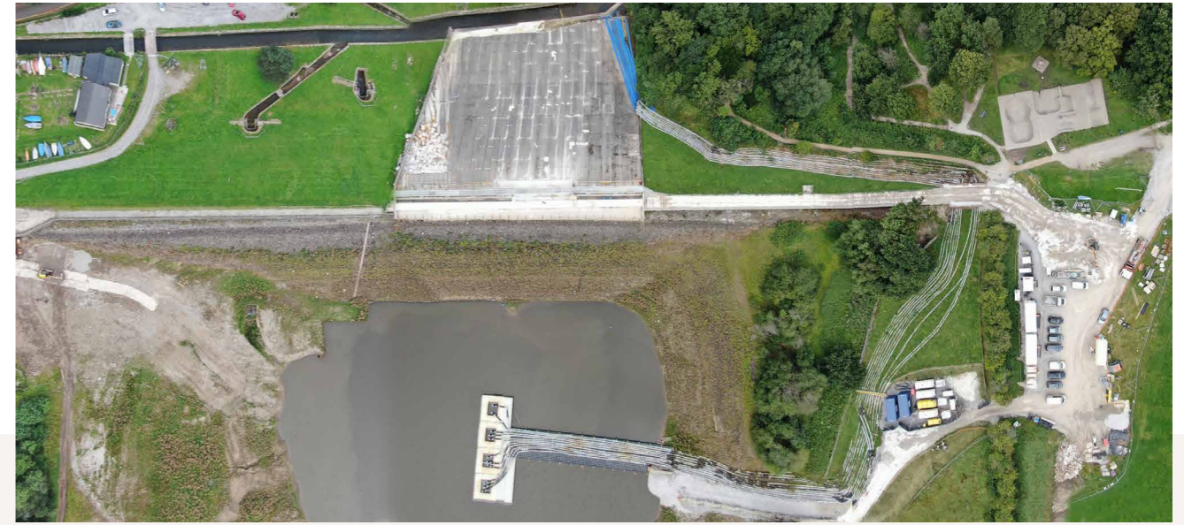
An aerial photograph of Toddbrook Reservoir and existing auxiliary spillway
