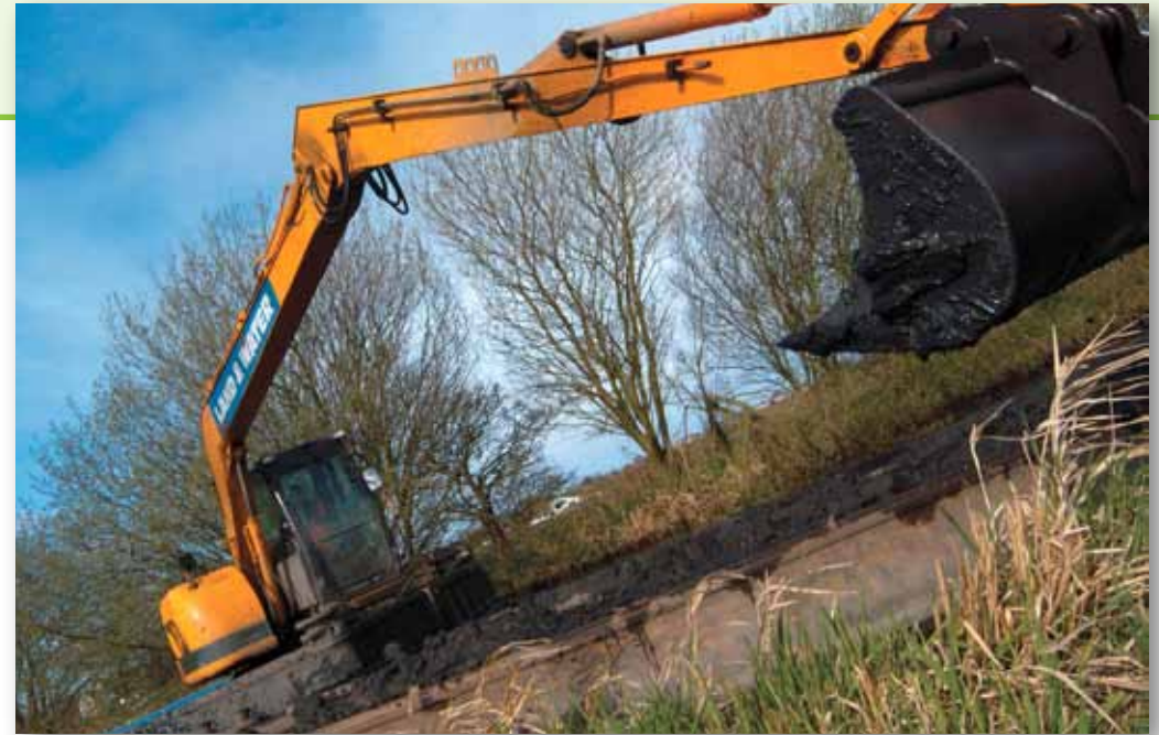
This dredger is removing mud from the bottom of the canal and putting it into a boat, called a mud hopper, to be taken away
