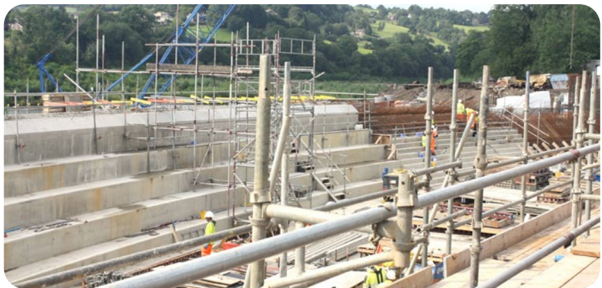
A new side weir and tumble bay are being constructed next to the reservoir at the top of the spillway. This will channel excess water from the reservoir into the River Goyt when the restored reservoir is full.
