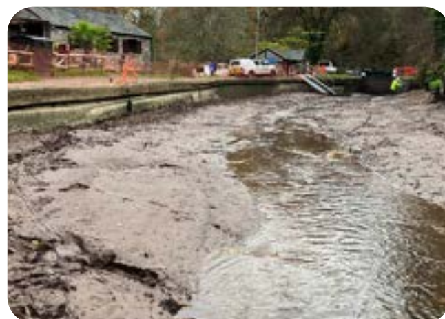
Above: Llangynidr Lock Flight on the Mon & Brec drained for repairs.
