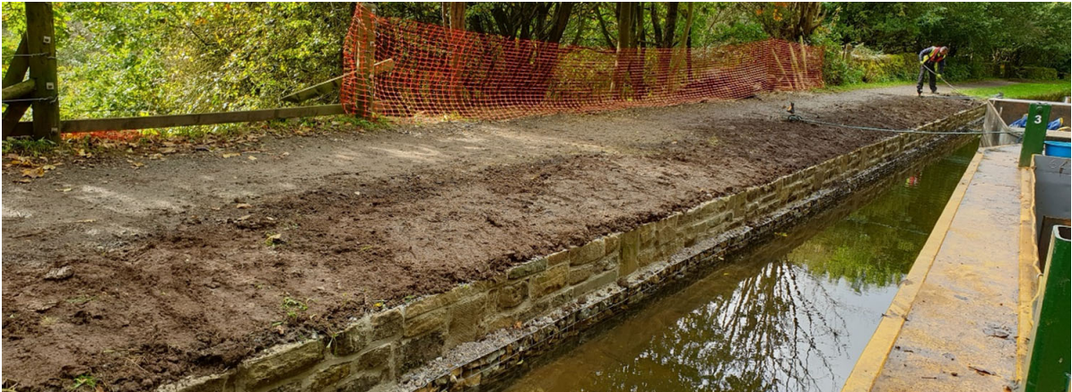
Tenterfields on the Rochdale Canal showing the completed waterway wall repairs
