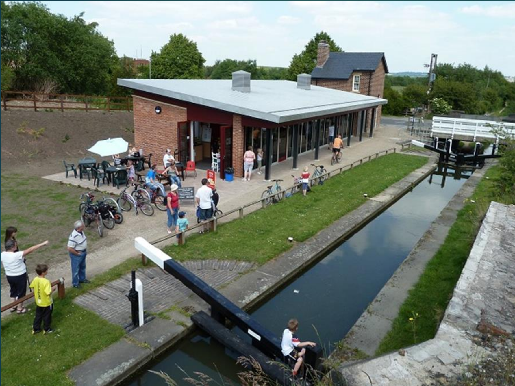
Hollingwood Hub, Staveley
