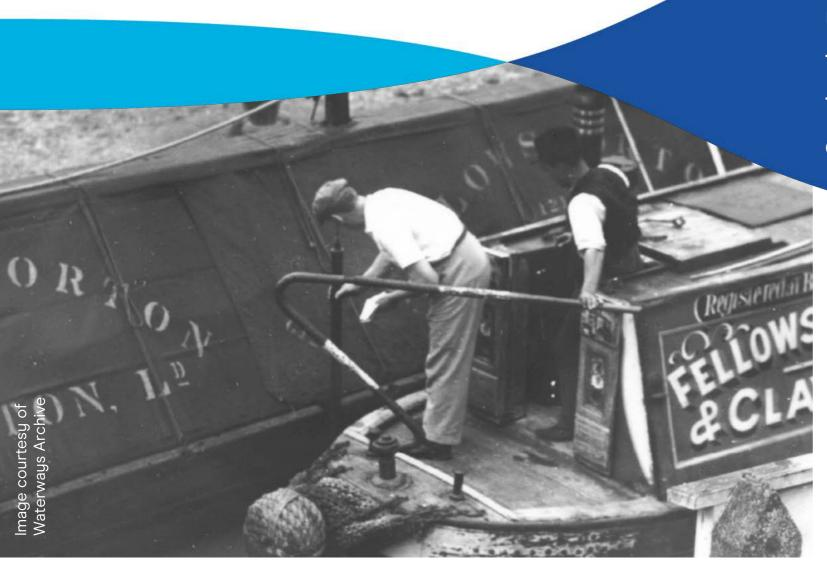
This picture shows a toll clerk using a gauging rod to measure the freeboard at set points around the canal boat, enabling them to calculate the toll to be paid.
