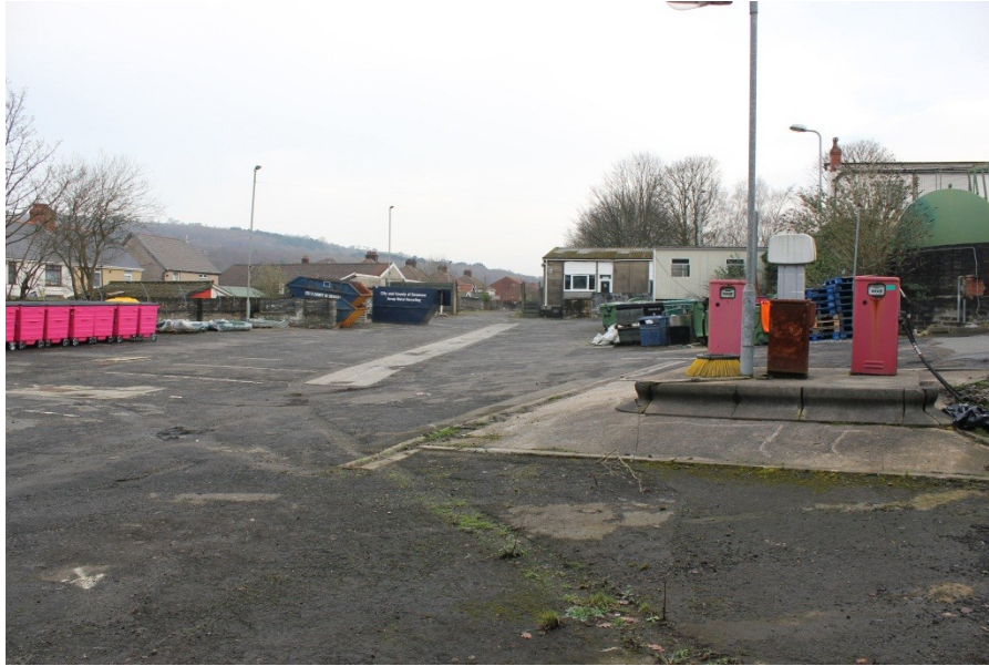
Image 1: Depot over canal line at Clydach
