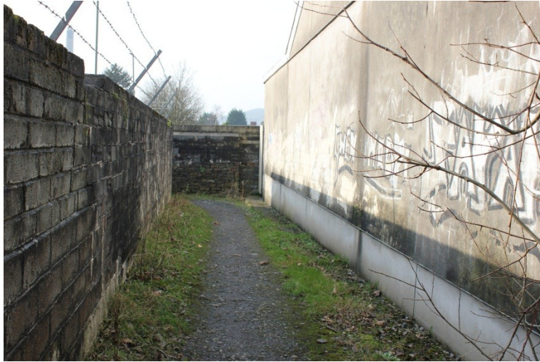
Image 13: The footpath linking the two lengths of canal at the depot
