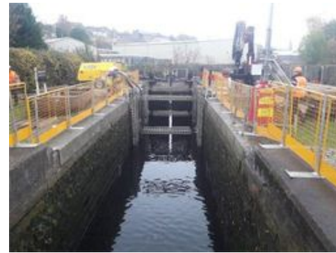
Battyeford Lock Stoppage – bottom gate replacement and brickwork repairs – Calder & Hebble Canal
