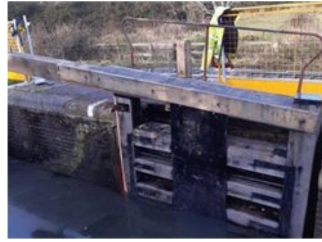
Aylesbury Arm Stoppages – Lock 2 bottom gate and Lock 3 top gate replacements
