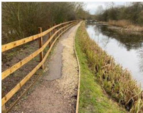
Towpath resurfacing work at Foxton
