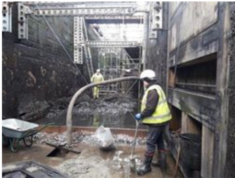
Battyeford Lock Stoppage – bottom gate replacement and brickwork repairs – Calder & Hebble Canal
