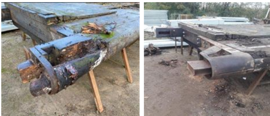
Stoke Bruerne Lock 14 Emergency Gate Repairs, GU Canal
