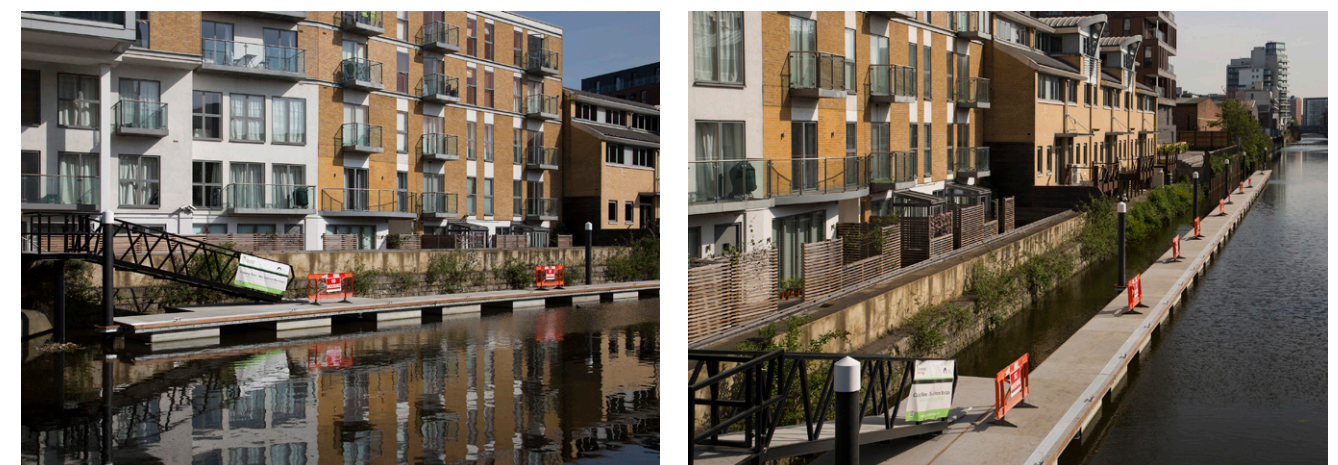
Photos of the mooring pontoon and bridging deck installed at Burdett Road.
