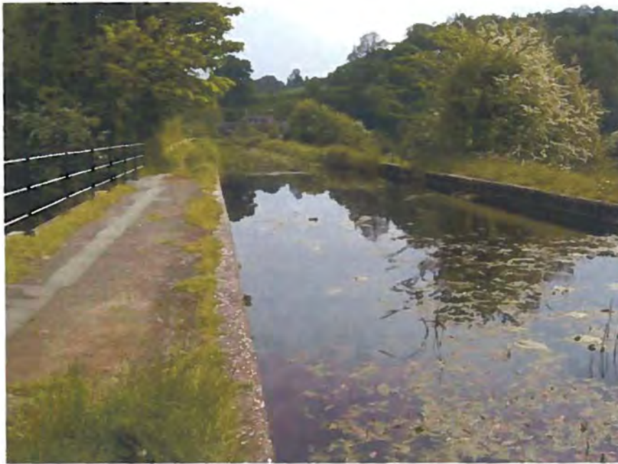
Figure 4.9 Aqueduct in the Montgomery Canal
