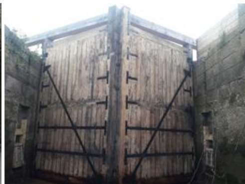
Tarleton River Lock 8 – New sea gates and paddles installed
