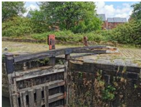
Emergency works to Lock 52 Rochdale Canal replacing broken balance beam
