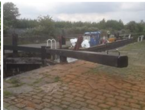
Emergency works to Lock 52 Rochdale Canal replacing broken balance beam
