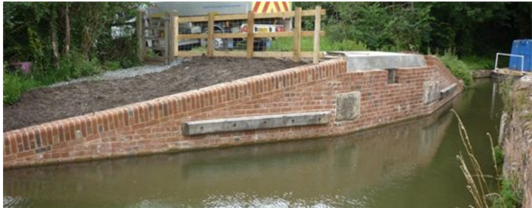
Reconstruction of offside wall at Drinkwater Lift Bridge, Oxford Canal, completed
