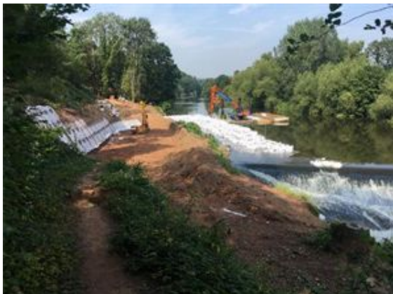
Holt weir - Temporary dam construction & soil nailing
