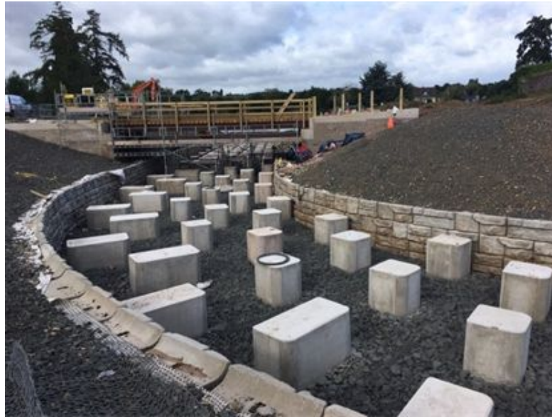
Bevere Fish Pass nearing completion
