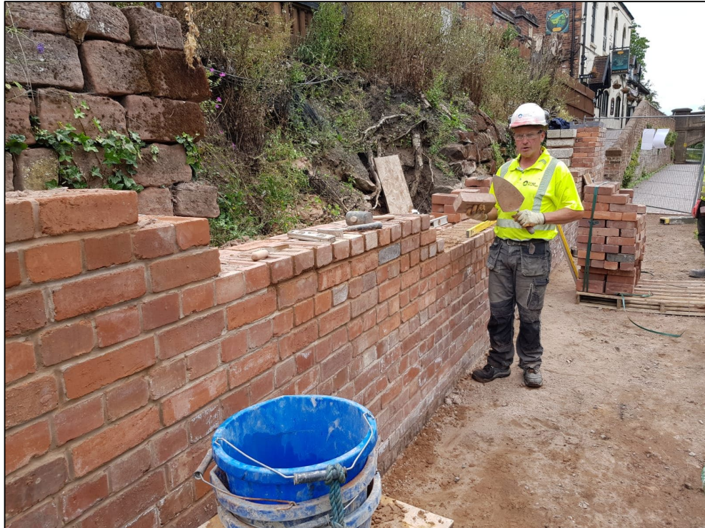
Black Star retaining wall rebuild on the Staffs and Worcester Canal
