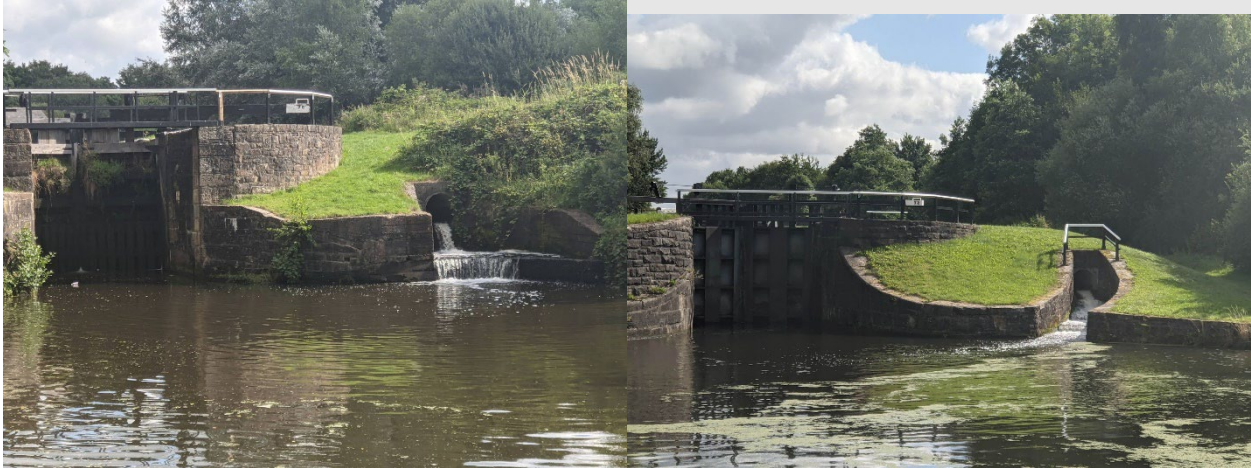
Headwall protections vs none.
