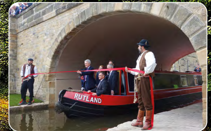
The bridge was rebuilt using modern civil engineering techniques, it kept its character with every numbered brick from the original put back in its place.
