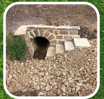
The failed culvert that caused the breach is now repaired and as good as new
