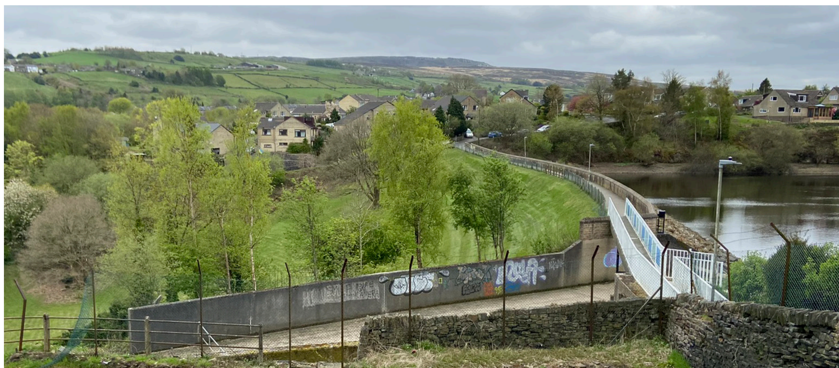
Photograph of the current spillway.
