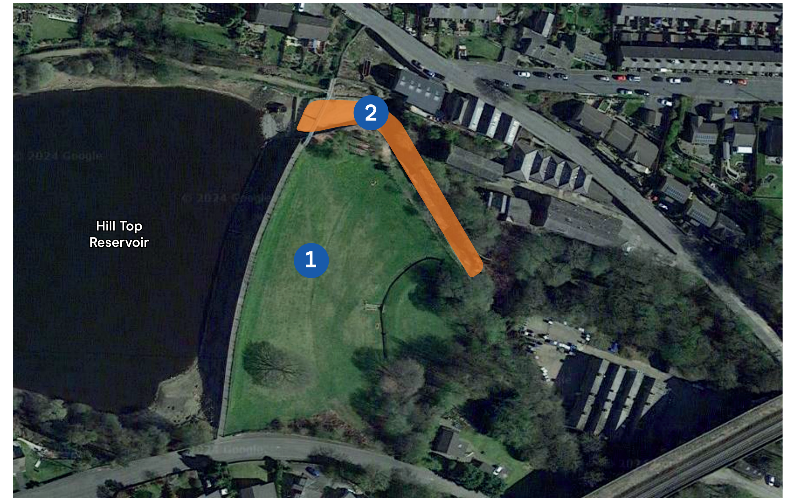
Key features of work (Courtesy of Google Maps).
