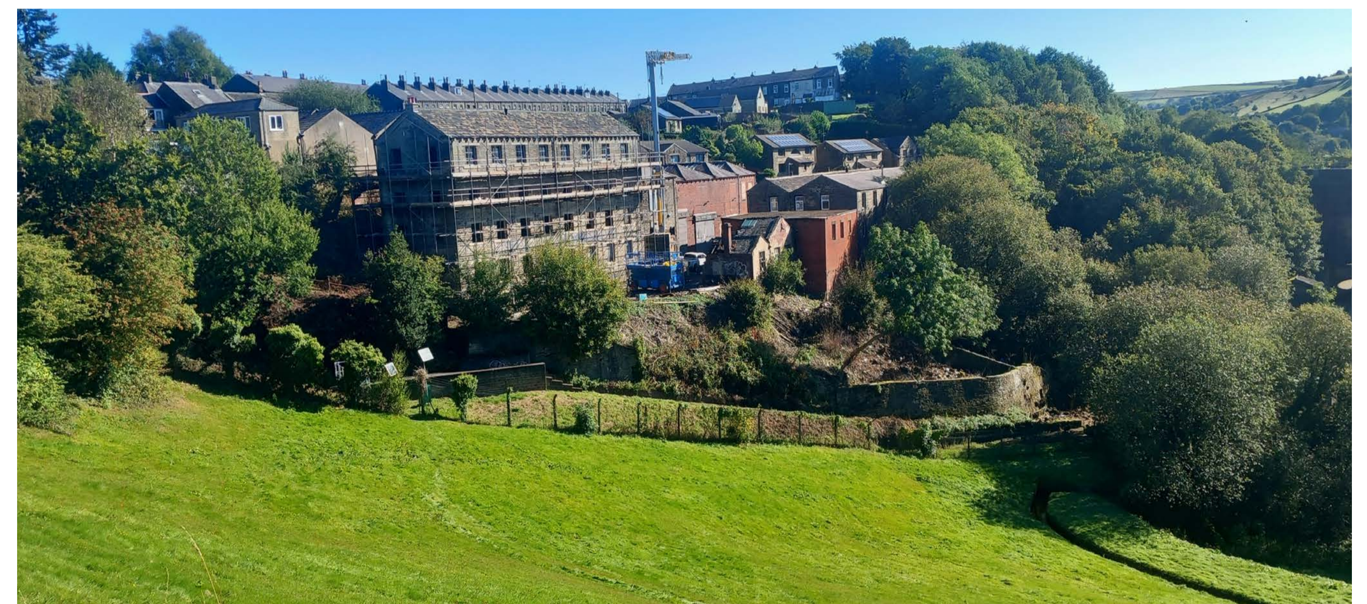
Photograph showing the current view of the spillway from the footpath at the crest of the dam.
