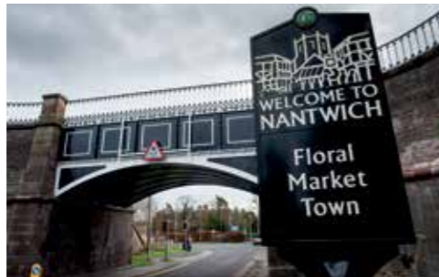
Community fundraising to repair Nantwich Aqueduct, Shropshire Union Canal
