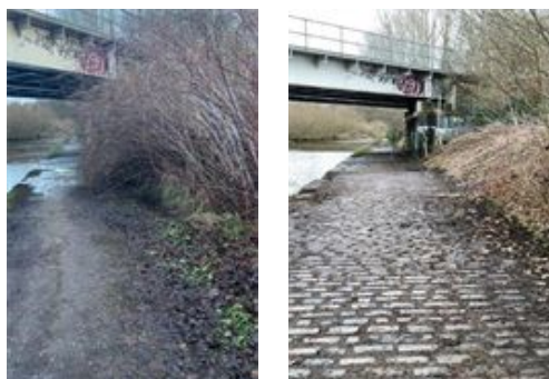
Before and after photos of clearance work on the Rochdale Canal
