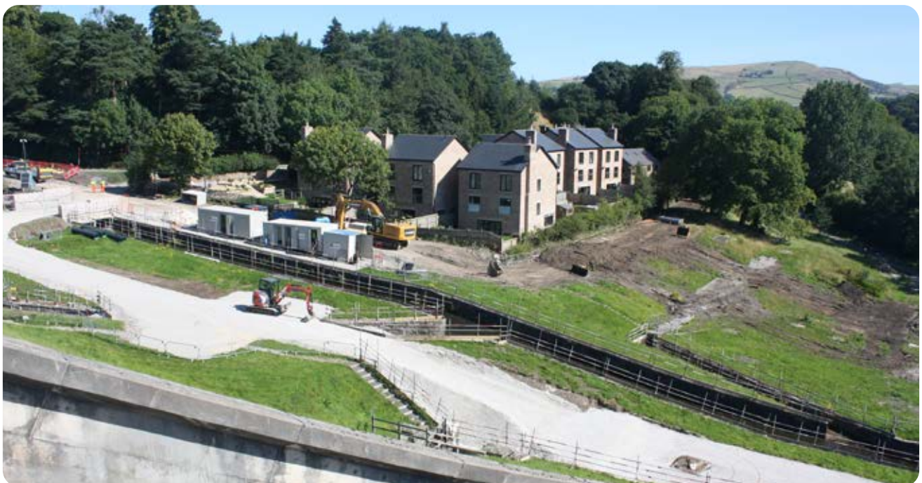
Above: Preparatory construction works include setting up a site compound and the diversion of drainage and feeder channels to make way for the new spillway.
