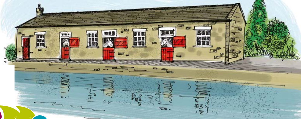
The Stables at Bingley Five Rise Locks
